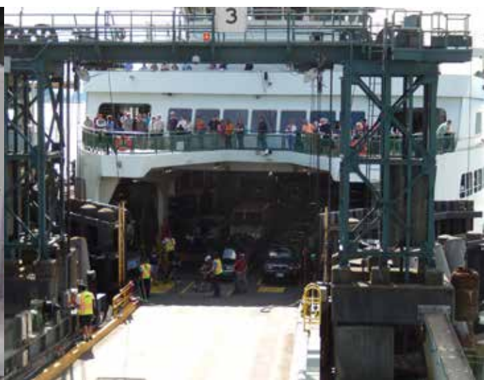
Washington State Ferry Terminal
